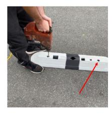
Drill two guide holes using base as a template.
