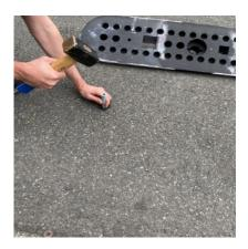
Use a hammer to place the two plugs into the holes.
