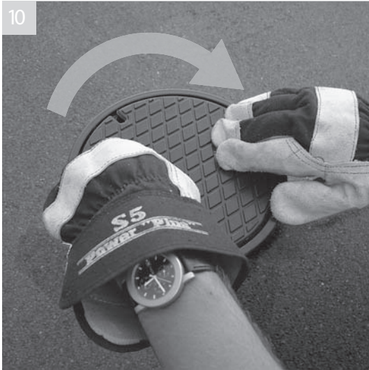
Twist blanking cap clockwise until lock is heard to engage
