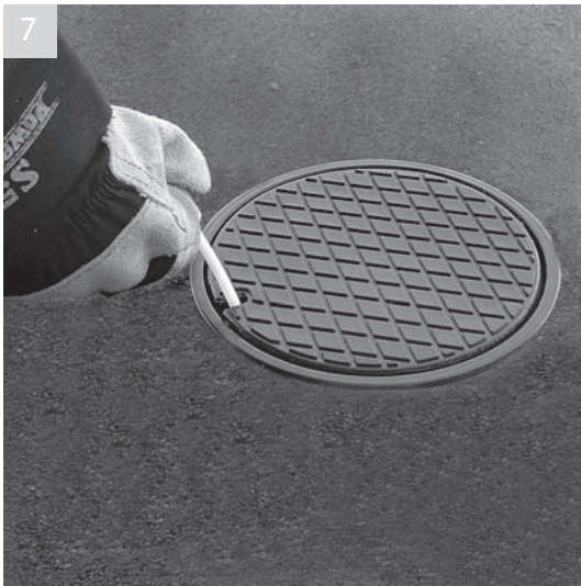
Insert key rod into key hole angling the key inwards so that the tip of the key is pushing against the socket stem
