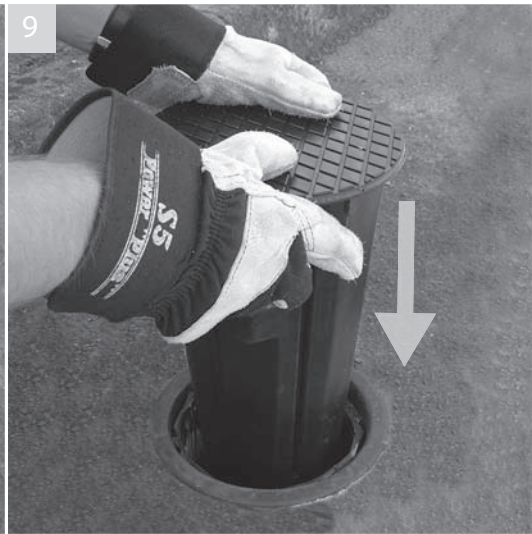
Replace blanking cap aligning horizontal locking pin in socket with the deep groove in blanking cap
