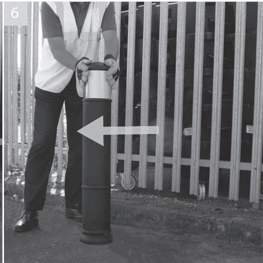
Twist bollard clockwise until lock is heard to engage
