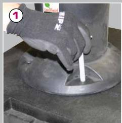
Ensure supporting course is no less than 100mm in depth. Position bollard and mark through the holes with chalk.
