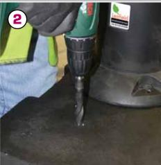
Drill 15mm holes at the four marked positions to a depth of 115mm to accommodate the ground fixing bolts.
