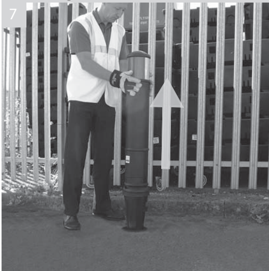
Lower bollard into socket
