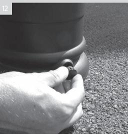
Replace plug. Repeat steps 10 - 12 removing the plug from the opposite side of the bollard
