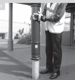
Slide bollard over steel core to ground level. If fitted with reflective banding orientate so that red faces into the direction of trafic flow
