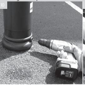
With bollard at final resting level remove one 6mm hole through the steel core
