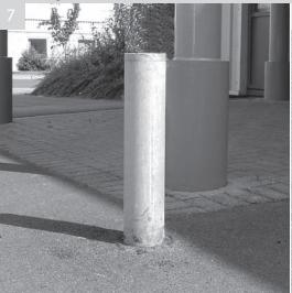
When concrete has cured replace final wearing Equally space the three spring clips around course to ground level
