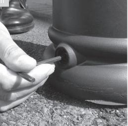
Using allen key screw in a grub screw through plug. Using bollard screw port as a guide drill a the threaded port in the bollard and into the core
