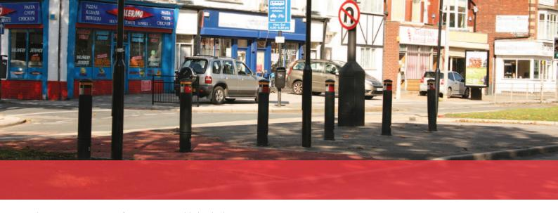
Thus in an emergency, fire engines could slowly drive over the bollards and they would then bounce back to upright preventing right turns for the general public. They approached Leafield Environmental to determine a fixing method that would allow the bollard to be easily replaced if broken in this process and a socketed version was developed for this purpose.
